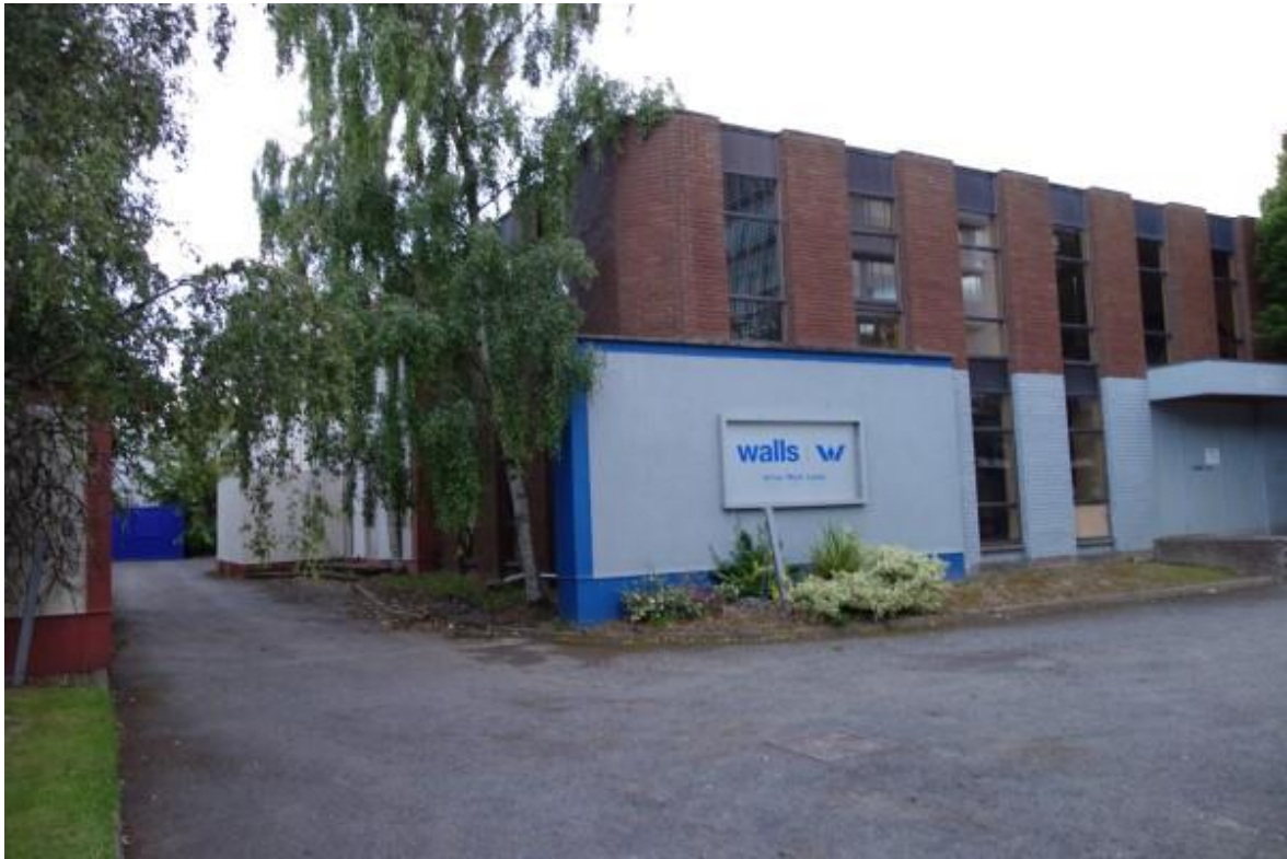
Figure 1: Northern side of main warehouse
