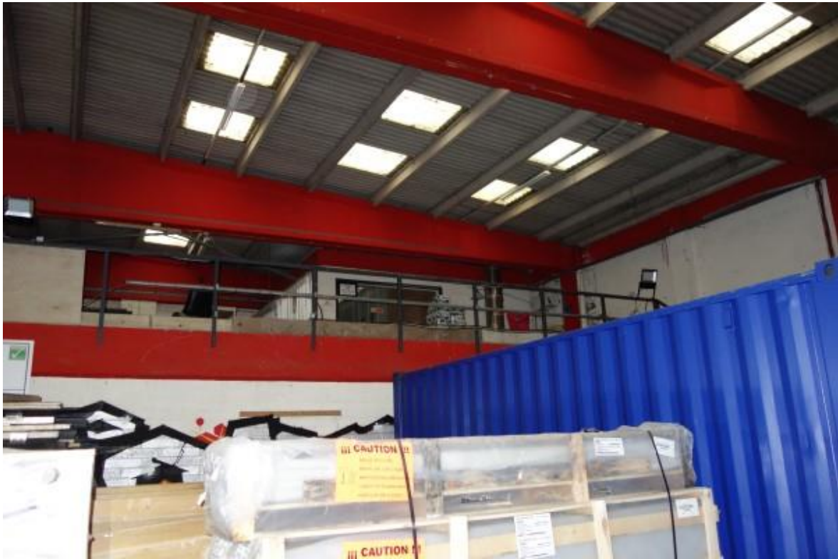
Figure 2: Interior of main warehouse
